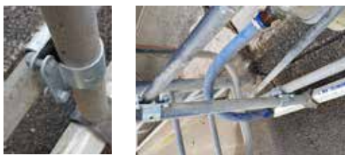
Normal clamps attachment of slider pipe to backing gate
