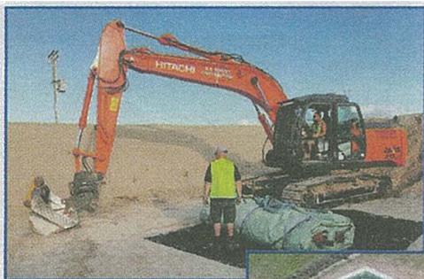
Groundwork and installation of the Ecobag underway.
