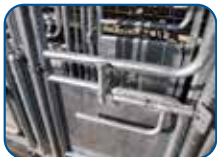
STEEL GATE PANELS Welded to frame.
