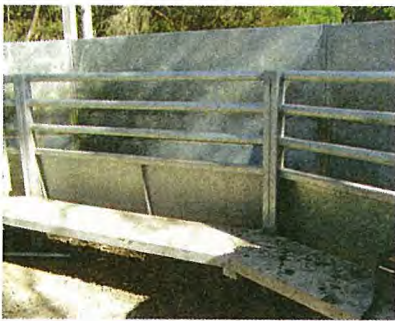
A non-slip concrete catwalk beside the race.
